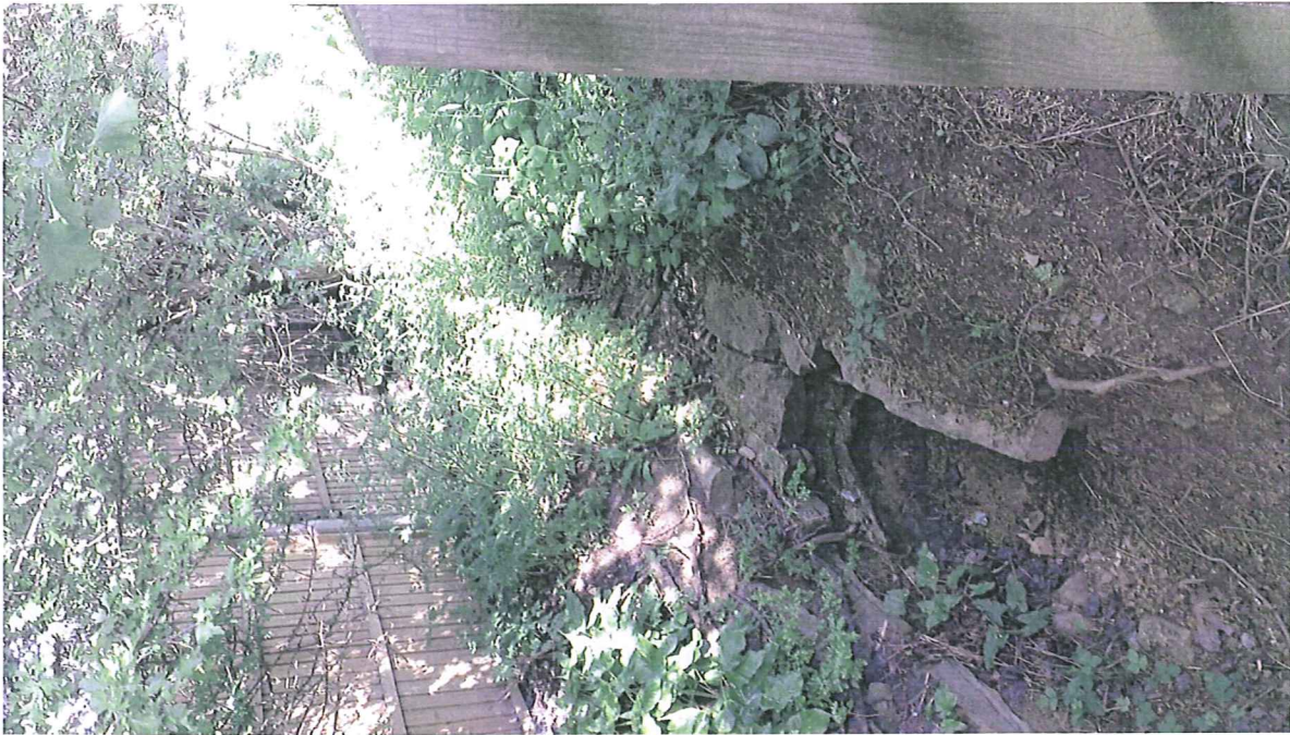
Photo E -- View upstream of Photo D Culvert
